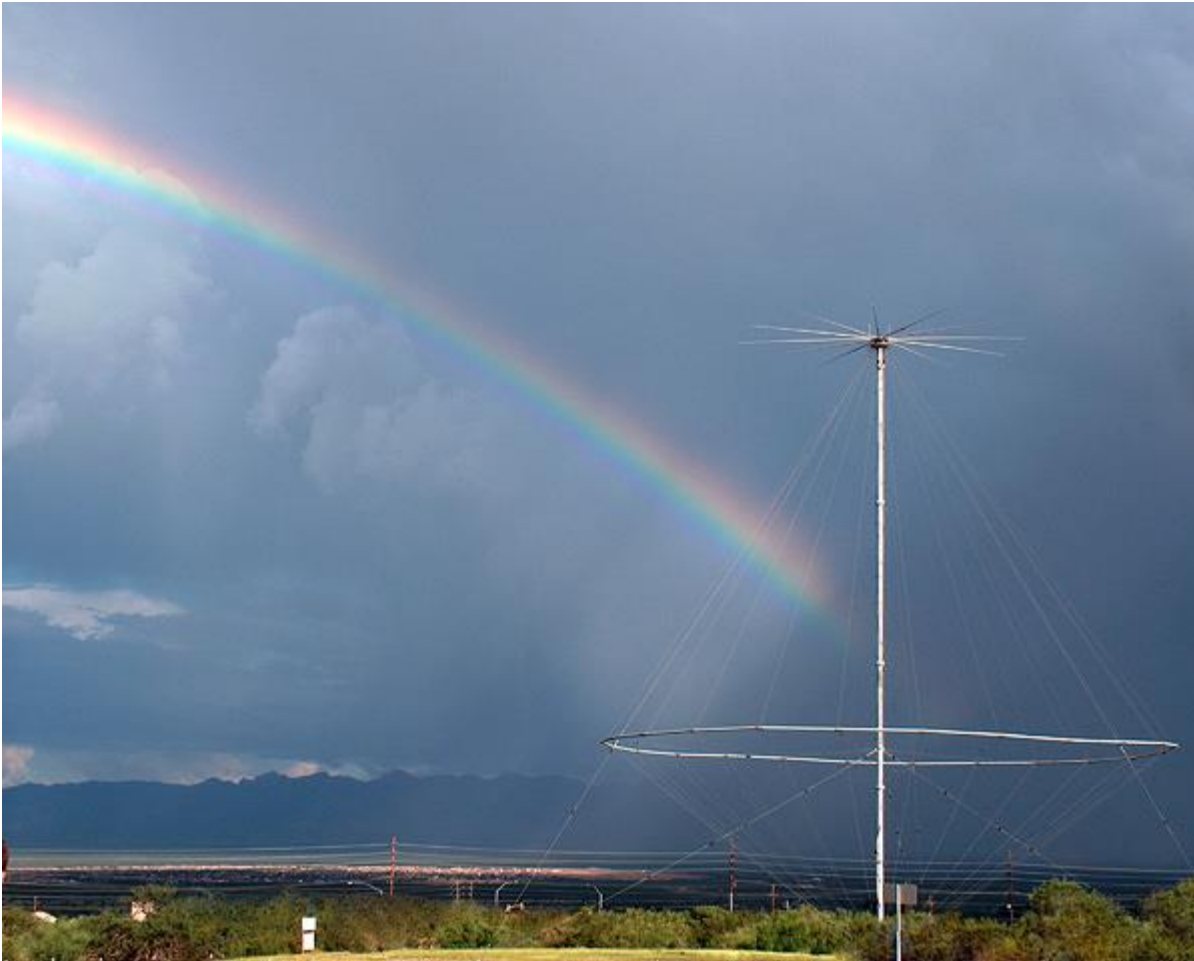
GVARC Full Band HF Discone Green Valley, AZ 80 feet
